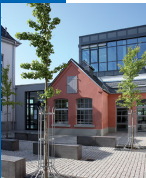
Innenhof Campus Erbenheim
